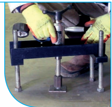
It is vital to establish substrate anchorage ability before installation
