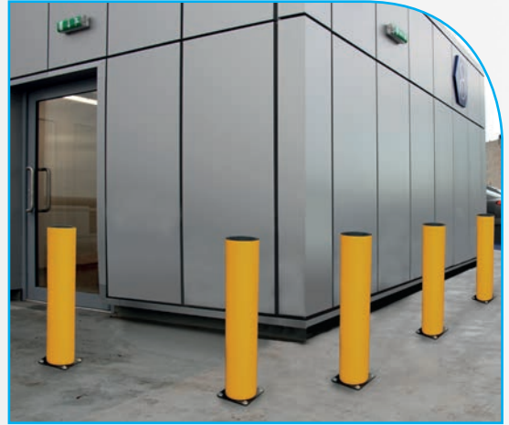
Bollards - Stair Core Areas
