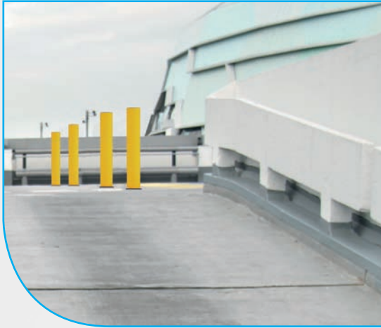
Bollards - End of Ramp
