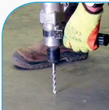
Testing substrate for compliance is essential
